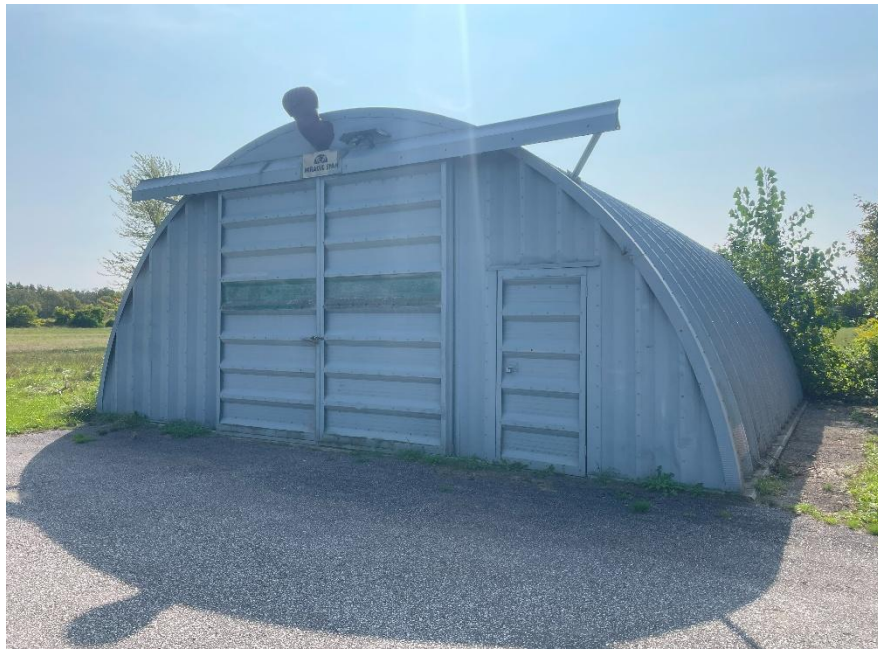
Photograph 3: View of existing storage structure (facing south) – September 9, 2025
