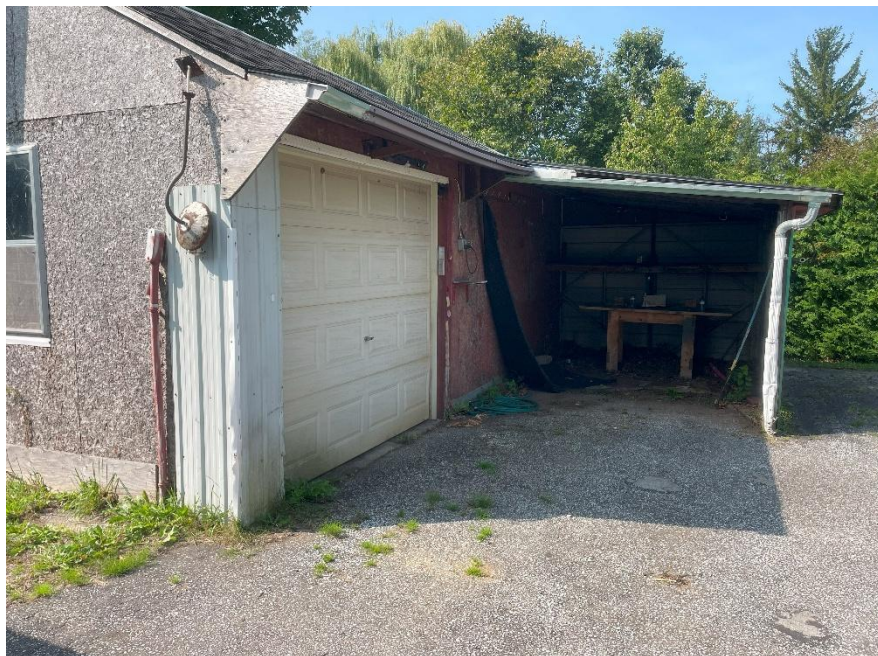
Photograph 4: View of existing storage structure (facing west) – September 9, 2025
